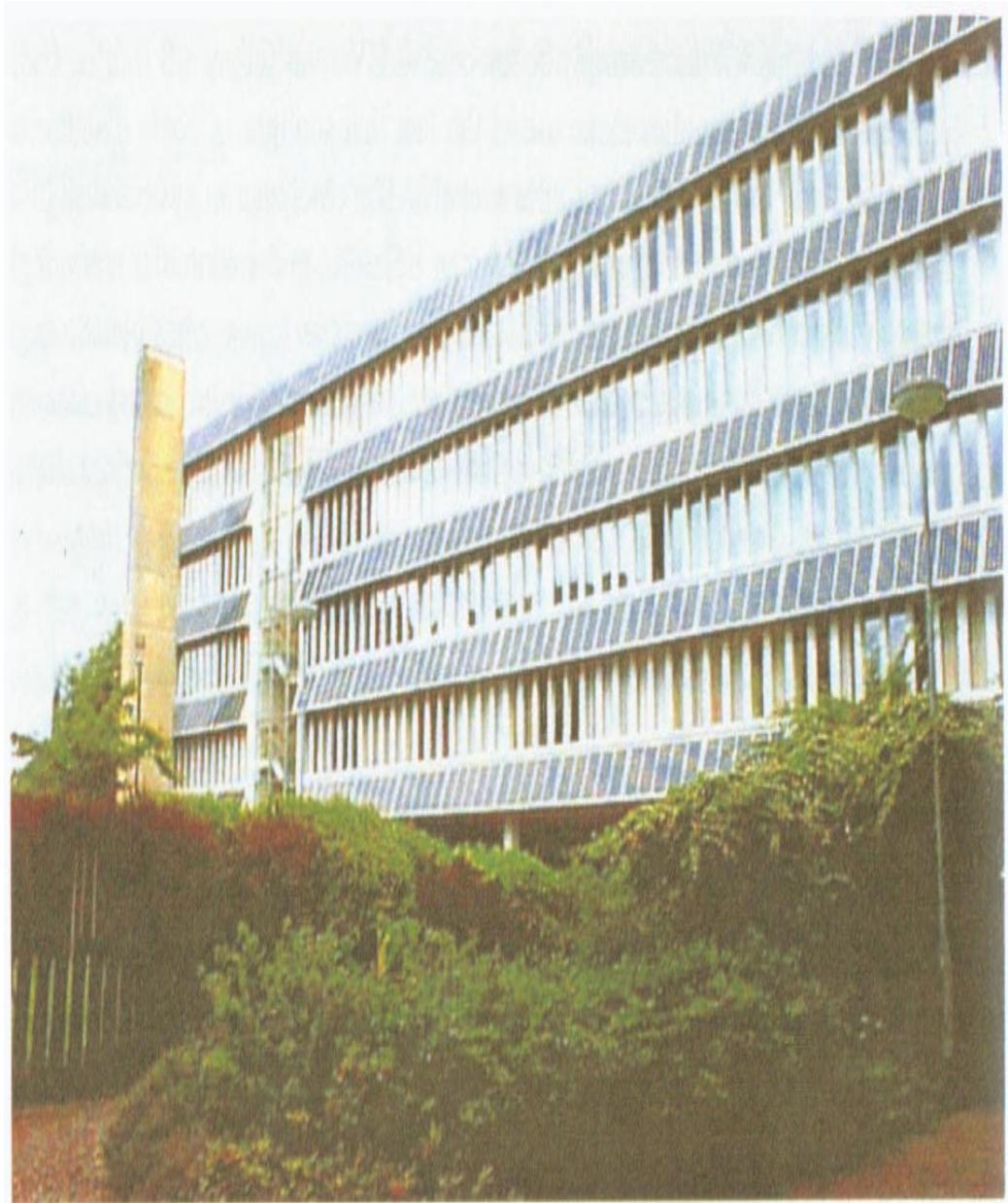
Figure 4.5 Example of façade integration of photovoltaics. The photograph shows the 40 kW<sub>p</sub> PV façade on Northumberland Building at the University of Northumbria. The PV array is integrated into the rainscreen overcladding. This system was installed in 1994 and is one of the early examples of façade integration (photograph courtesy of University of Northumbria).
