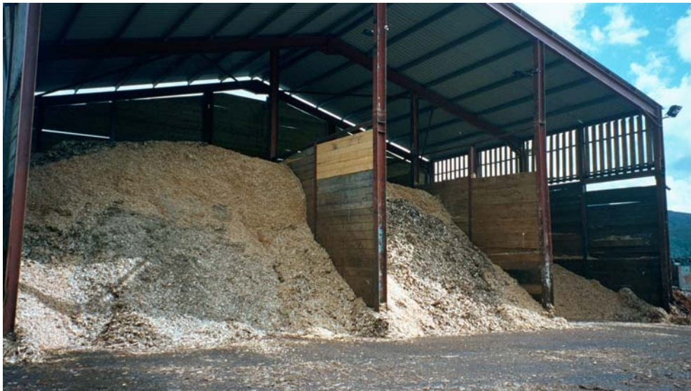
Figure 29 – Woodchip stores. The woodchips will eventually be used as fuel.
