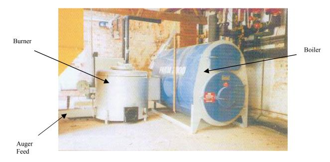
Fig. 32(a): A woodchip boiler system (pre-combustor design: see also 5.4.1.4) [23]
