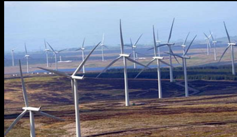
Whitelee Wind Farm, Scotland – UK’s largest with 215 Siemens and Alstom wind turbines and a total capacity of 539 MW (2017).
