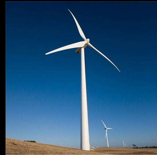
Vestas 2 MW wind turbine.
