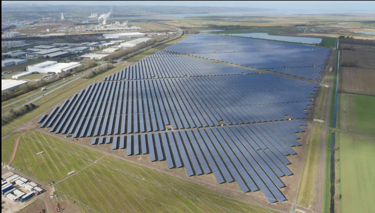
Shotwick solar farm – 72MWe
