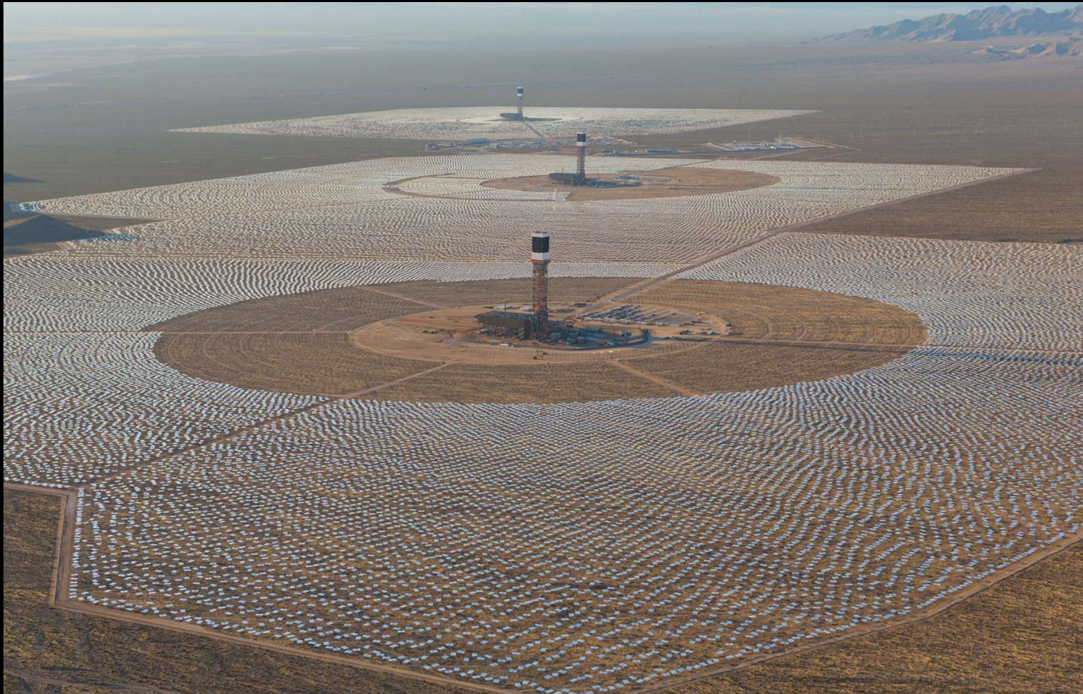
Ivanpah solar power plant, Mojave Desert California – 392 MW, 173,500 heliostats
