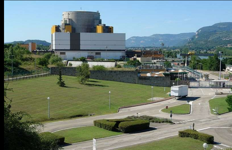
Superphénix in France (1984-1998), at 1200 MWe, the largest FBR yet built.
