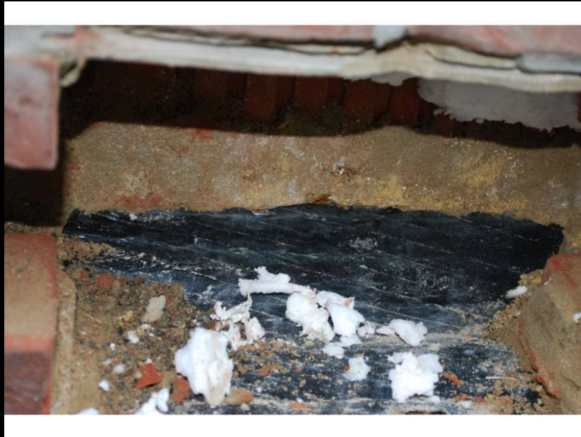
Cavity tray wrongly detailed.
