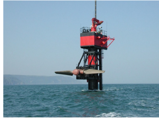
300 kW horizontal-axis turbine
