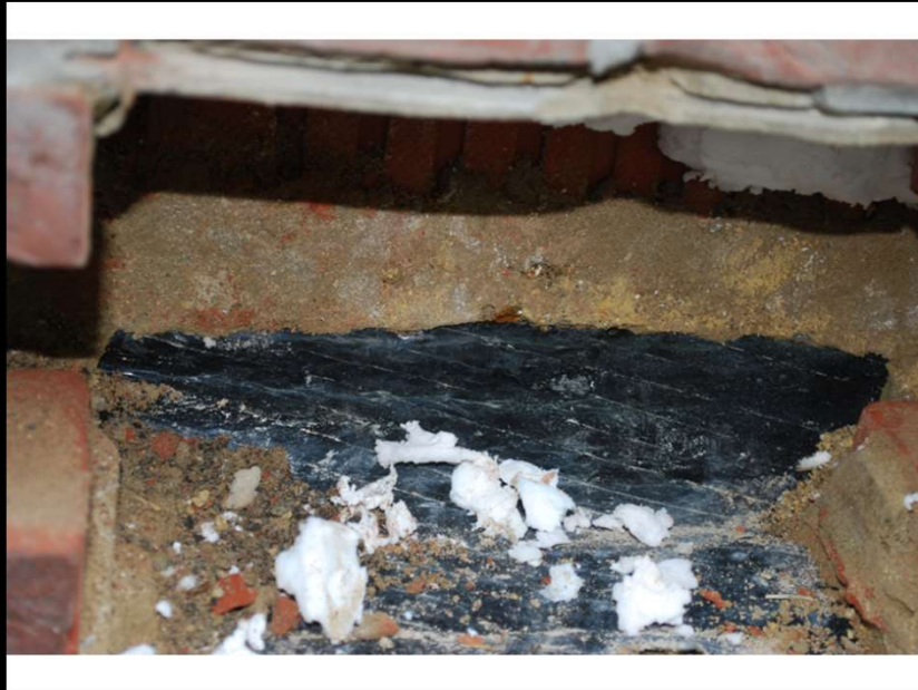
Cavity tray wrongly detailed.
