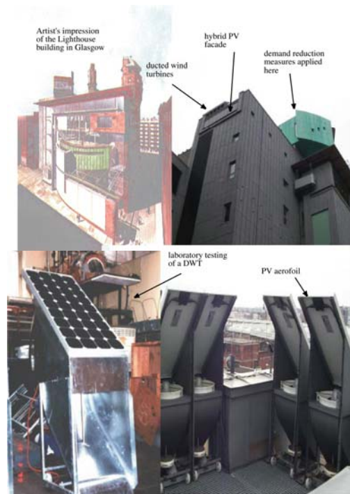
Figure 3: Renewable energy components as incorporated in the Lighthouse building in Glasgow.
